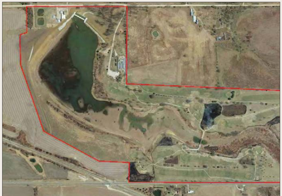
This aerial view of the Osage City Lake from Google Earth shows the nearly empty condition of the lake in March of 2014. The red boundary shows the approximate extent of the City of Osage City property. Much of the exposed lake bed shown in this photograph was dredged.
